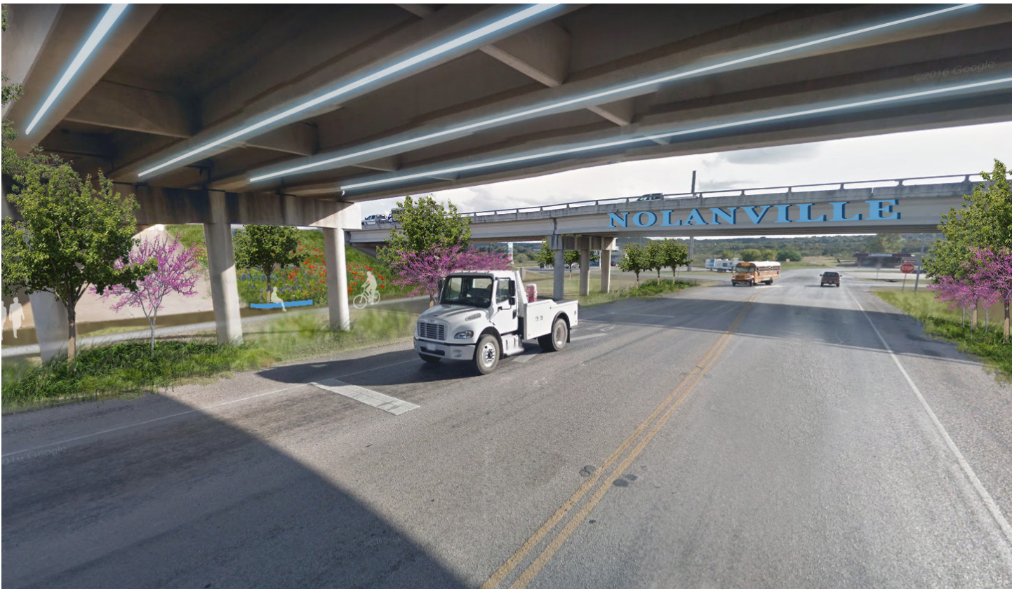
View Beneath Overpass
